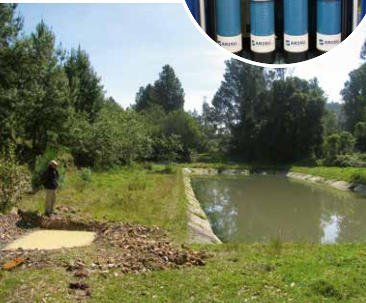
The water situation in San Miguel before the project
