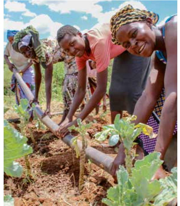
Installation of irrigation systems
